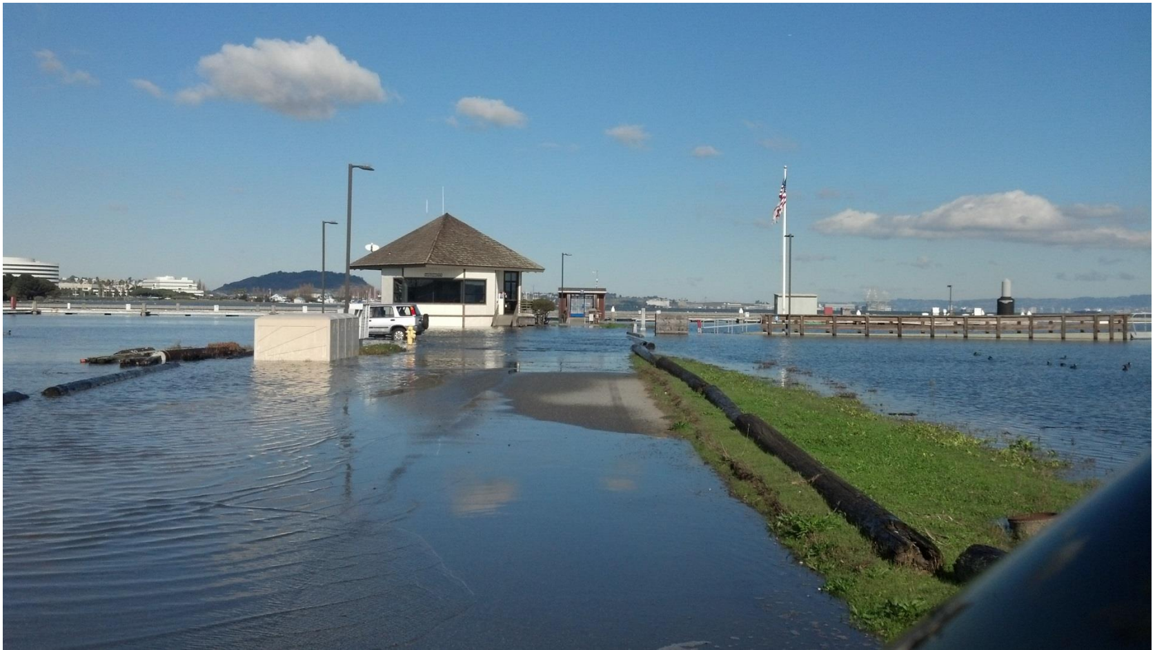
Oyster Point Marina Harbor Office and King Tides
