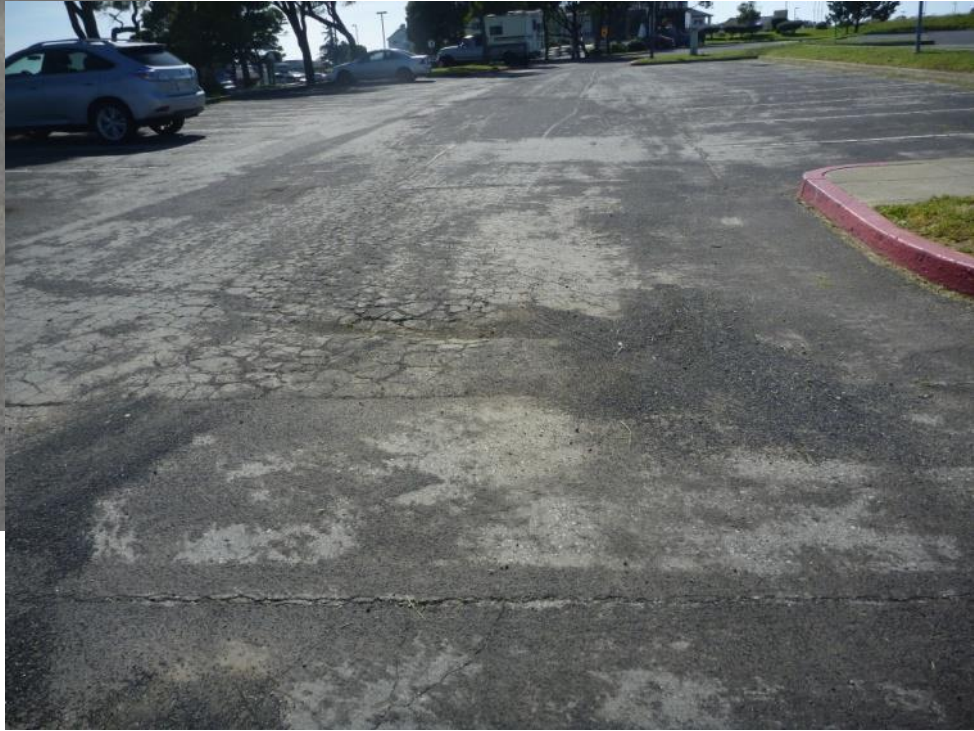
Roadways at Pillar Point Harbor
